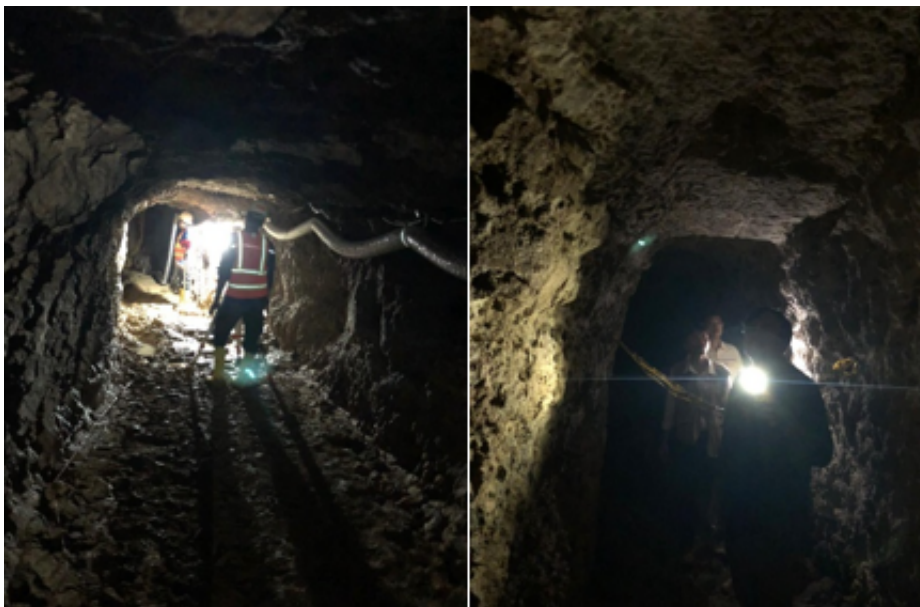
Figure 2. The condition of the opening hole is relatively damp
