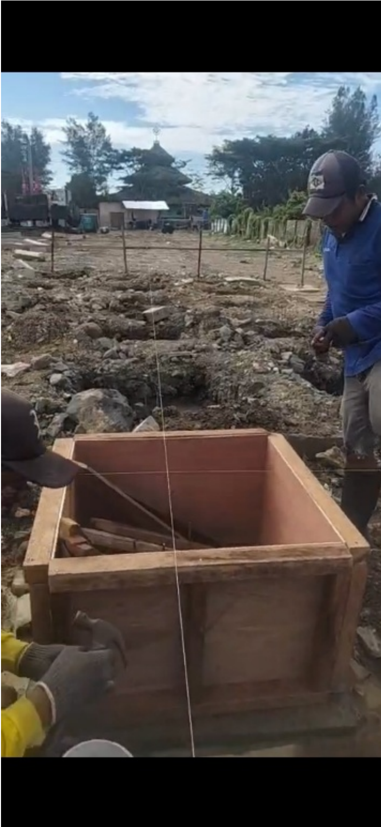
Figure 10. 10 Pemasangan Bekisting PC2
