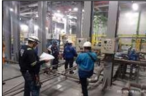
Gambar 3.11 Inspection Marine System
