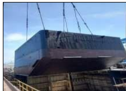
Gambar 3.10 Loading Block for Erection 206 S BMPP
