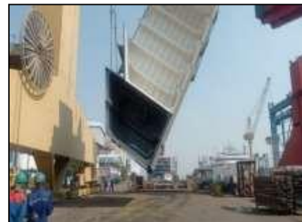
Gambar 3.9 Proses Loading Block 206 C BMPP
