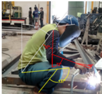
Figure 2. Pengelasan Platform Catwalks
